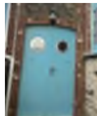
Right: The new doors fitted at the back and front doors
